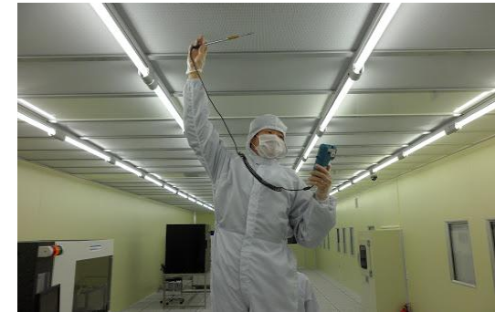
Clean room & UT Hook-up
