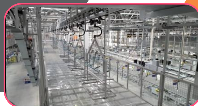
OHC (Over Head Conveyor)
